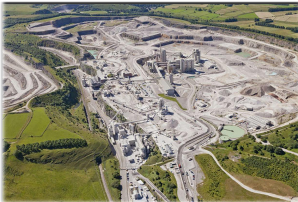
Plate 3-2: Existing Tarmac Tunstead Cement Works
